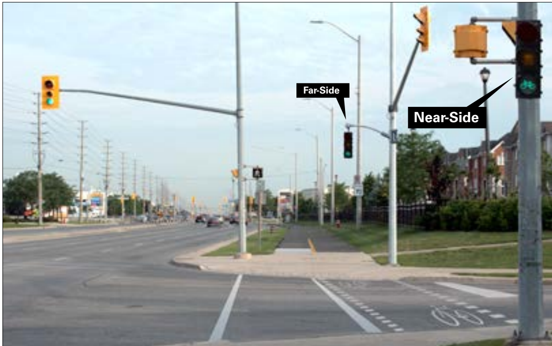
Figure 18 – Image: Multi-Use Trail Beside Traffic Signal, Signal Control, Crossing Configuration A, Near-Side/Far-Side
