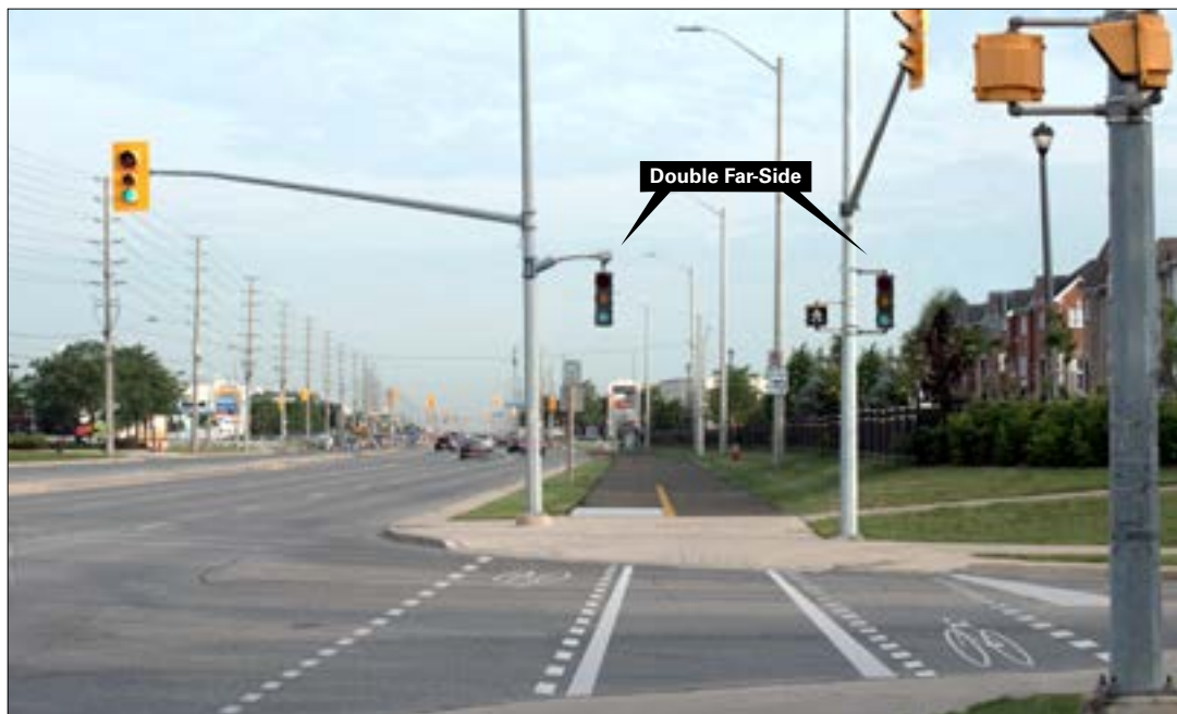
Figure 17 – Image: Multi-Use Trail Beside Traffic Signal, Signal Control, Crossing Configuration B, Double Far-Side
