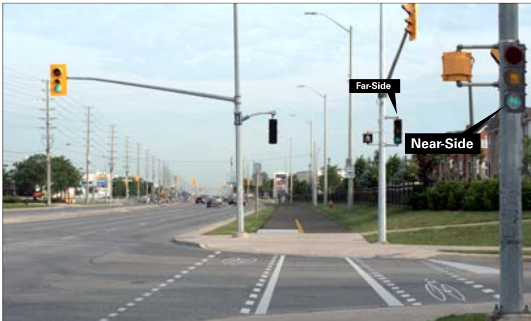
Figure 16 – Image: Multi-Use Trail Beside Traffic Signal, Signal Control, Crossing Configuration B, Near-Side/Far-Side
