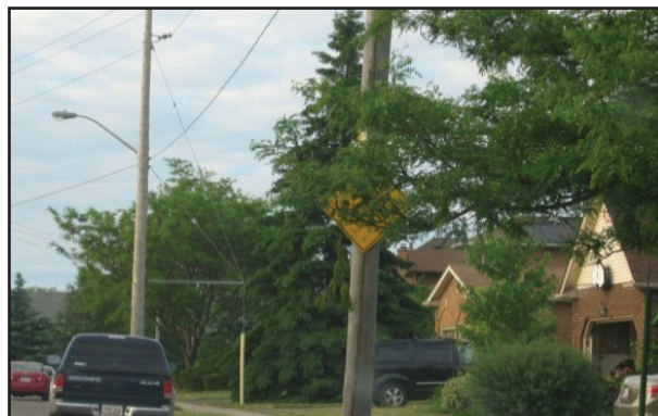
Vegetation control maintenance required.
