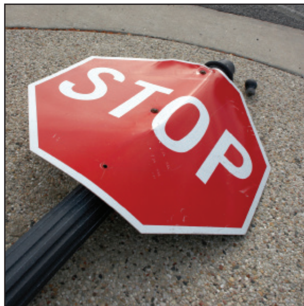
A fallen stop sign requires emergency maintenance.
