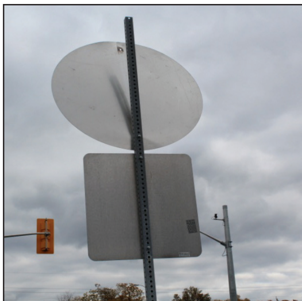
New, no heavy truck sign. The top fastener on the “new” sign has failed. Planning is required to determine whether the sign fasteners should be replaced or if the “new” portion of the sign can be removed.
