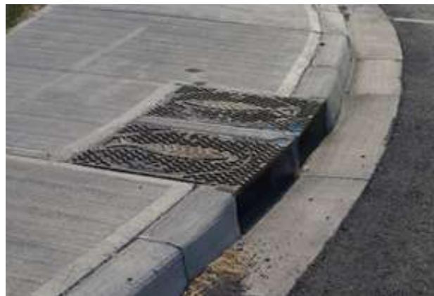
Figure 7.15 – Side-Inlet Catch Basin
