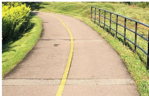
Figure 10.8 – Transverse Cracking
