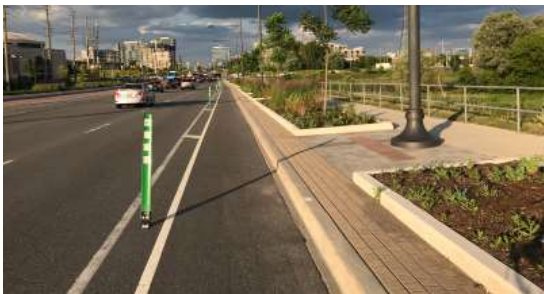
Figure 4.23 – Flex Bollard Separation, Markham
