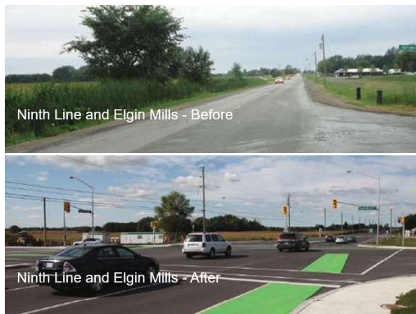
Figure 8.6 – Pre- and Post-construction Comparison
