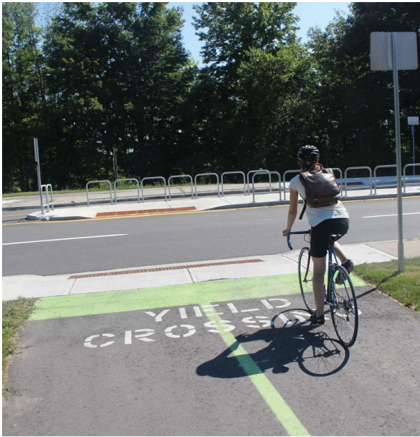
Figure 6.76 – Example of Uncontrolled Crossing, Toronto
