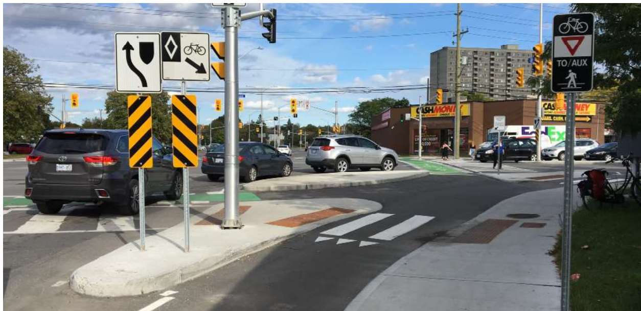
Figure 6.36 – Example of Protected Intersection Corner, Ottawa
