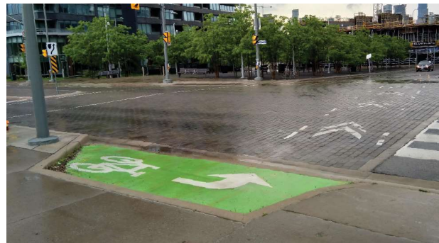
Figure 6.52 – Example of a Pocket at T-Intersection, Toronto
