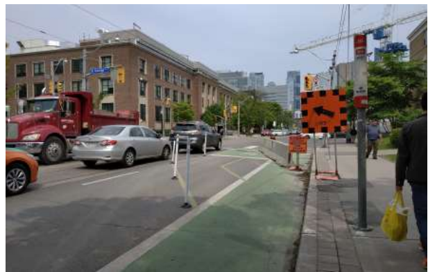
Figure 7.19 – Example of a Temporary Alignment for Physically Separated Cycling Lane, Toronto
