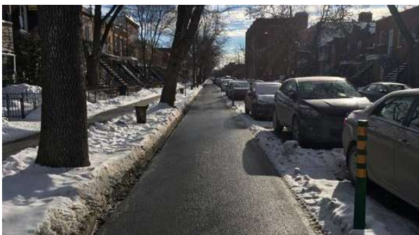
Figure 10.21 – Cycle Track Cleared by Sweeper with Brine Applied to Surface, Montreal
