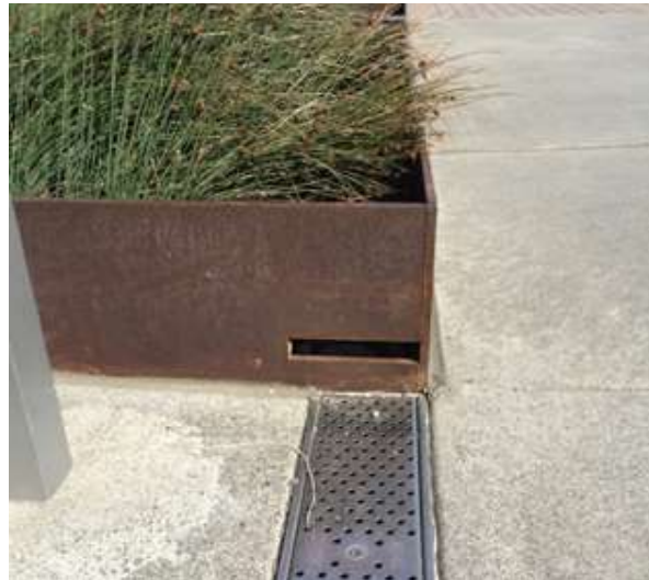
Figure 7.16 – Trench Drain at a Flush Surface
