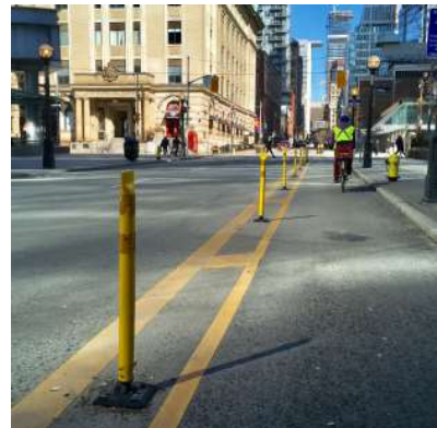
Contraflow Bicycle Lane Separated by Bollards, Toronto
