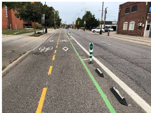
Figure 10.6 – Well-Maintained Cycling Facility, Hamilton
