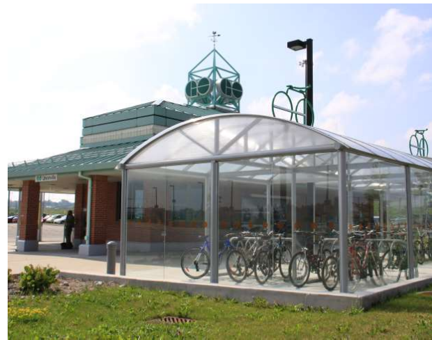
Figure 3.5 – Bike Parking at Commuter Rail Station, Markham
